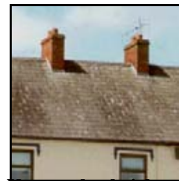
Vernacular brick chimneys
