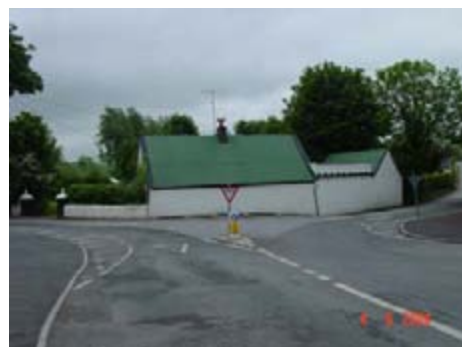
Junction at Village centre
