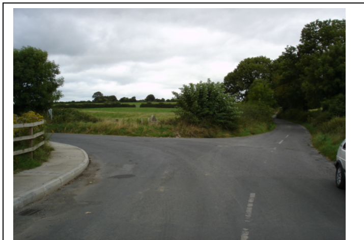
SO.9 Junction Improvements
