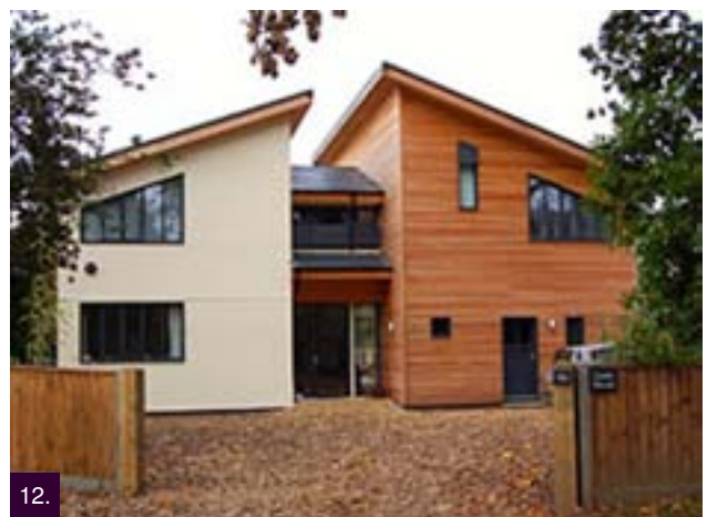
Award-winning family home based on sustainable design principles, including sheltered location, use of a ground source heat recovery system, high levels of thermal insulation, maximum use of natural lighting, and maintenance-free materials.
